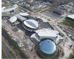
The impressive new headquarters of AFAS will consist of several buildings on of which will be a theater. The theatre is an eye-catching glass dome. Octatube was contracted to build this striking feature. The dome has a constant radius and is divided into several horizontal rings, which are divided by a triangular pattern. A dome is an efficient design feature in terms of the use of materials and the structural rigidity creates a lot of space.
